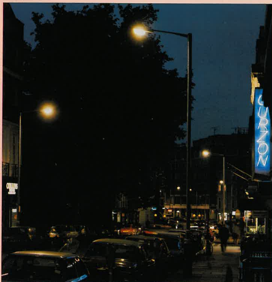
In Curzon Street, (below) existing lanterns originally housing 1,000W incandescent lamps were replaced by 400W SON, as were those outside the Horseguards in Whitehall shown above.
